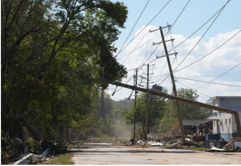
Photo 1. Infrastructure damage in Buncombe County, NC. Source: Madeleine Cook, Federal Emergency Management Agency, 2024
