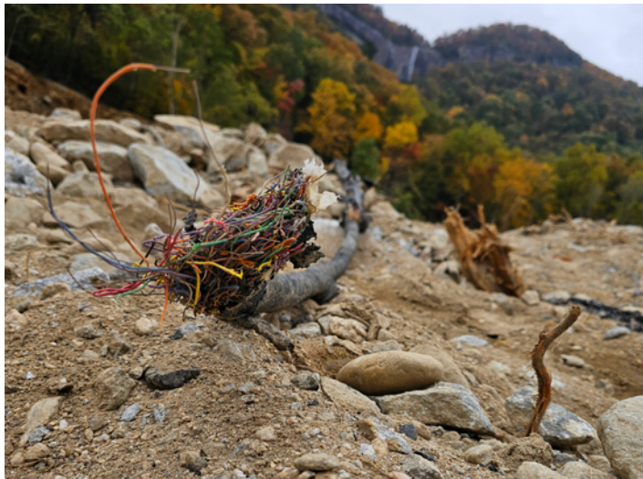
Photo 2. Severed telecommunication line at Chimney Rock debris field. Rodney Cooper, ITDRC.
