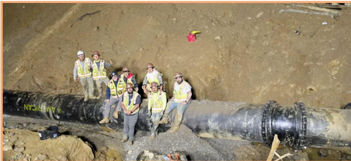
Figure 14. T and K Utilities crew connecting Asheville's water supply 53 days after Tropical Storm Helene (Photo Credit: Taylor Howard).
