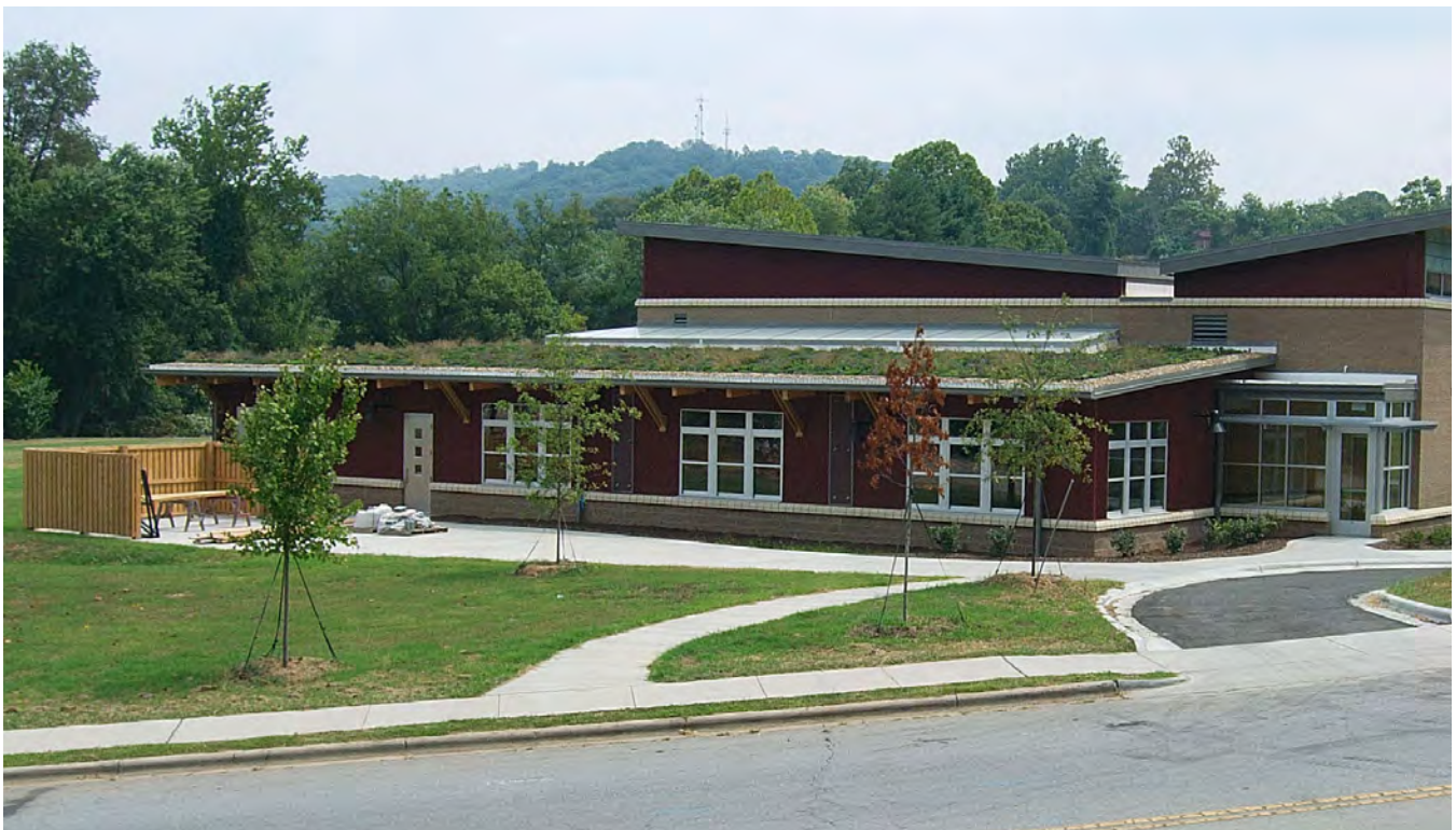
The green roof at the Dr. Wesley Grant Sr. Southside Community Center in Asheville.
