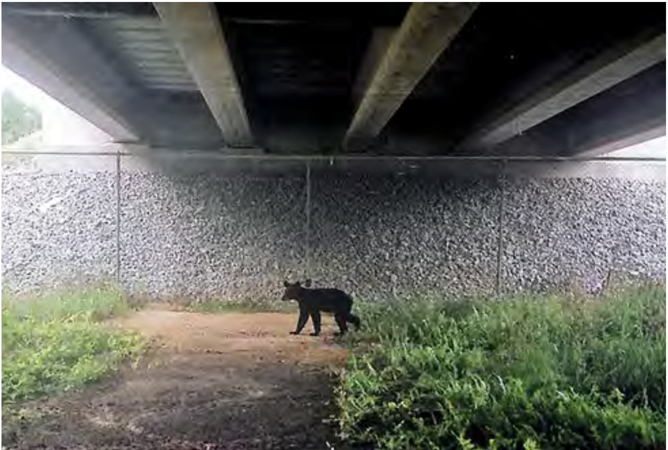
The first underpass wildlife crossings in North Carolina were built on a section of Interstate 26 in Madison County. The two 8 x 8 feet concrete boxes are primarily intended for use by North American black bears.
